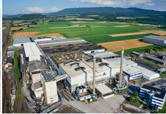
Pöchlarn Plant, Austria
